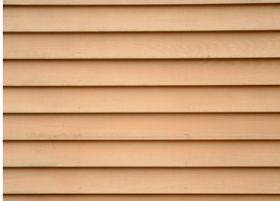
Exterior Wood Siding - Clapboard Wood Siding (2.5" Exposure) Color - SW 7004
